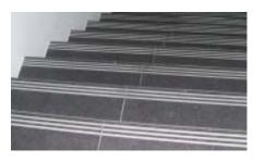
**Step Tread Grooves** By cutting grooves *into* the tile itself, a perfect non-slip stair nosing is achieved without sticking a self-adhesive grip strip (which has the potential to peel off over time).
