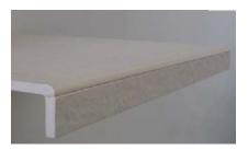
**Apron with Round Edge** The construction of this profile involves bonding a strip of tile (usually of 30 – 90mm height) at right angles onto the floor tile.
